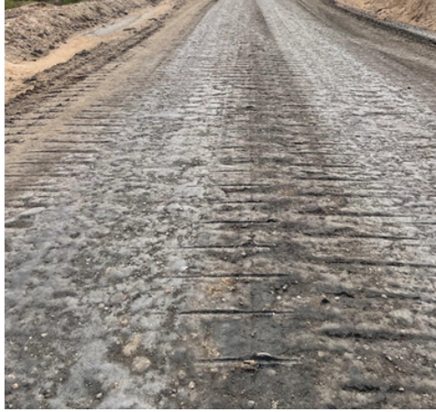
Figure 1. Example of an unpaved mining haul road exhibiting transverse irregularities and surface corrugation, which cause increased rolling resistance, fuel consumption, and maintenance requirements for haul trucks.
